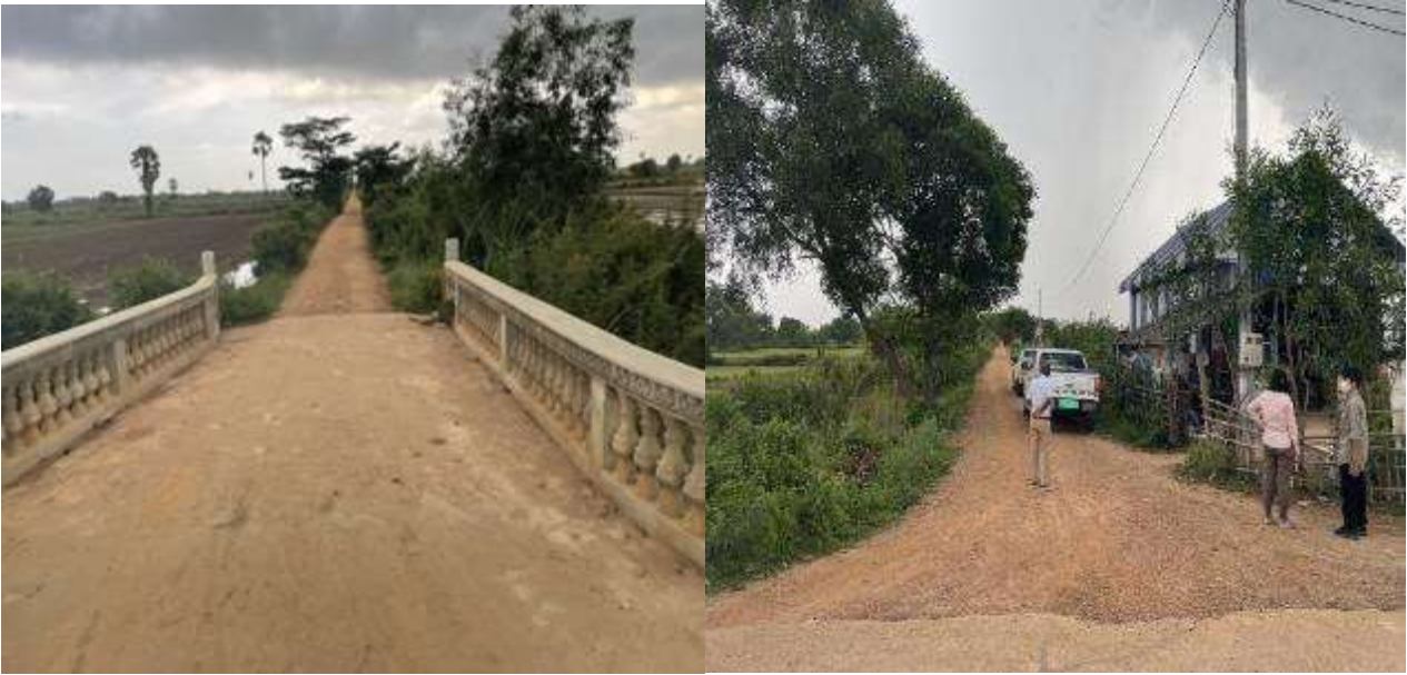
Figure 3: Original condition of road in So Sen commune
